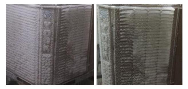
The images shown below is the beginning of the heat pump coil frosting due to normal operating conditions. Once the conditions meet the designed parameters of the defrost control board, the defrost cycle will be initiated.
