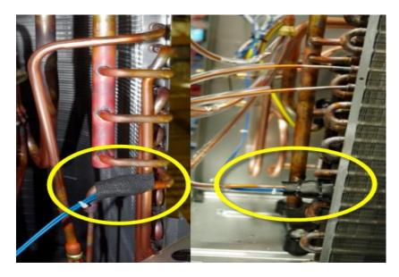
The images above illustrate the sensor at the bottom distributor line with a 3/8" stub for sensor (Thermistor) mounting.
